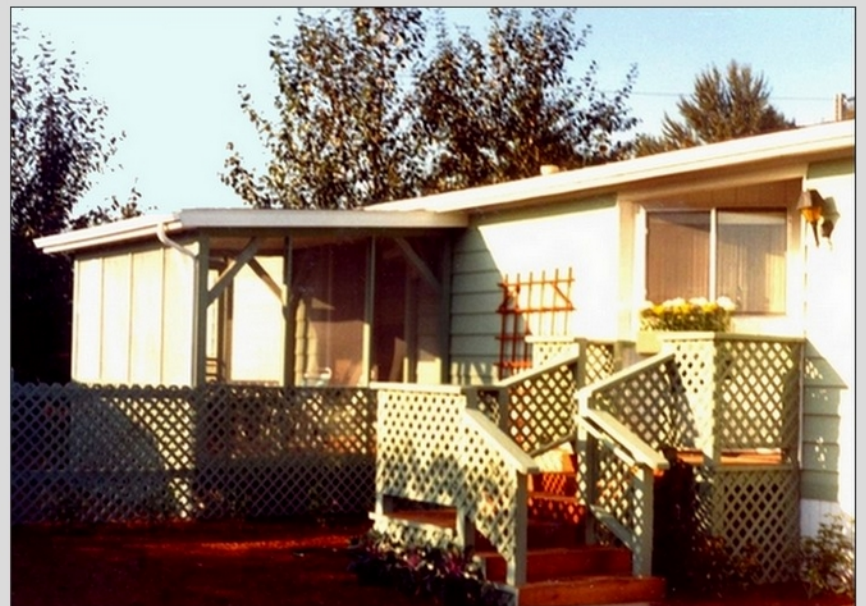
1988 - The finished porches
