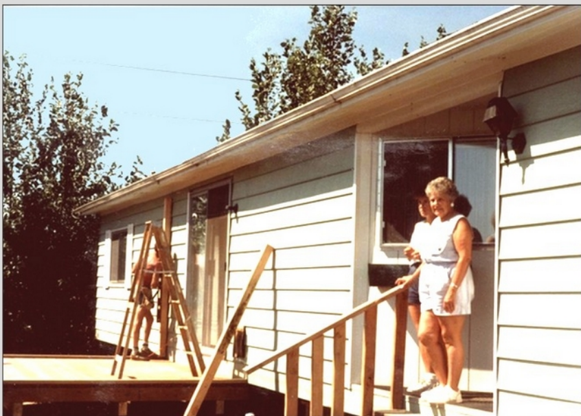
1988 - Building the porches
