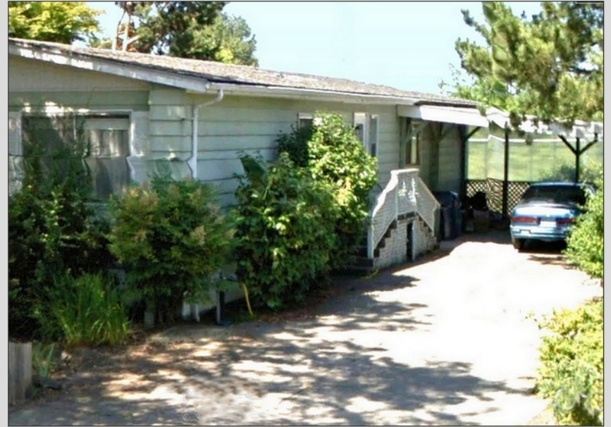
2011 - Back porch and carport
