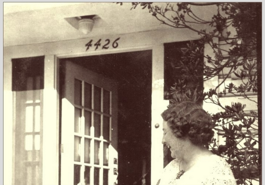
10th Avenue, front door
