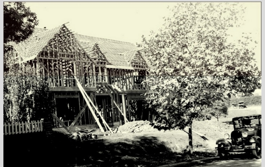
Forrester Drive, under construction
