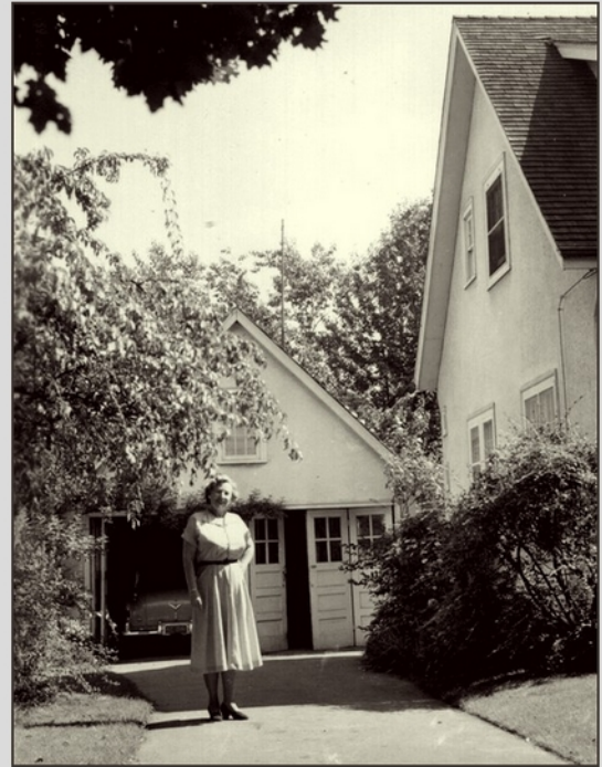
SE 34th Avenue, garage
