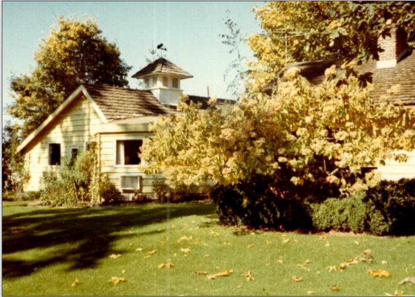
Peyton Road. garage from back
