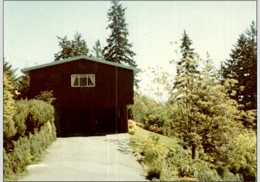
18th Place, garage and driveway
