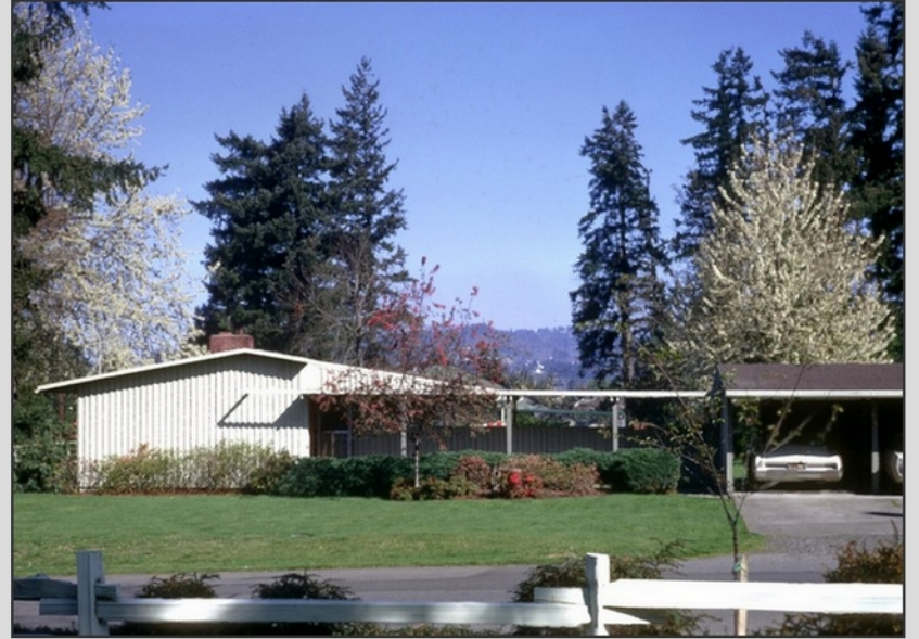
SW Peyton Road, from front yard
