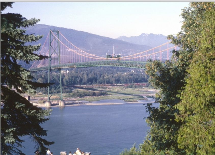
Lion's Gate Bridge, Vancouver, 1966
